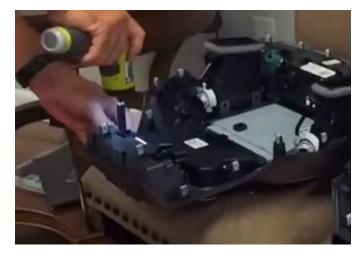
**Step 11:** Install the lower controls on to the new UAX Replacement Instrument Panel.
